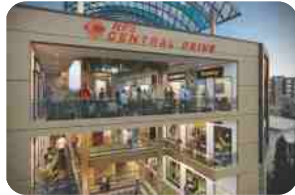
RPS Central Drive
