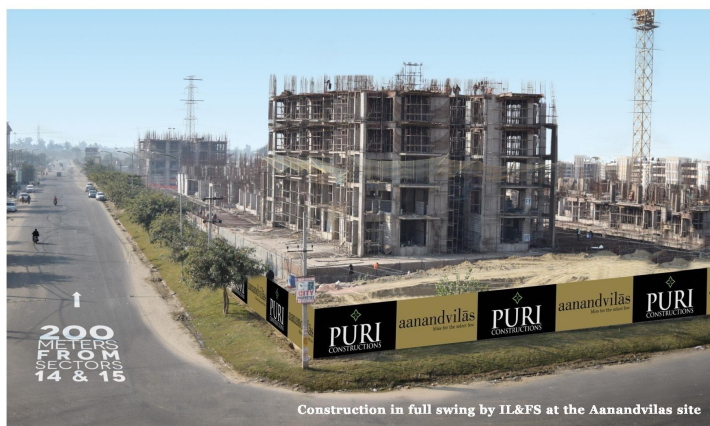
Construction in full swing by IL&FS at the Aanandvilas site
