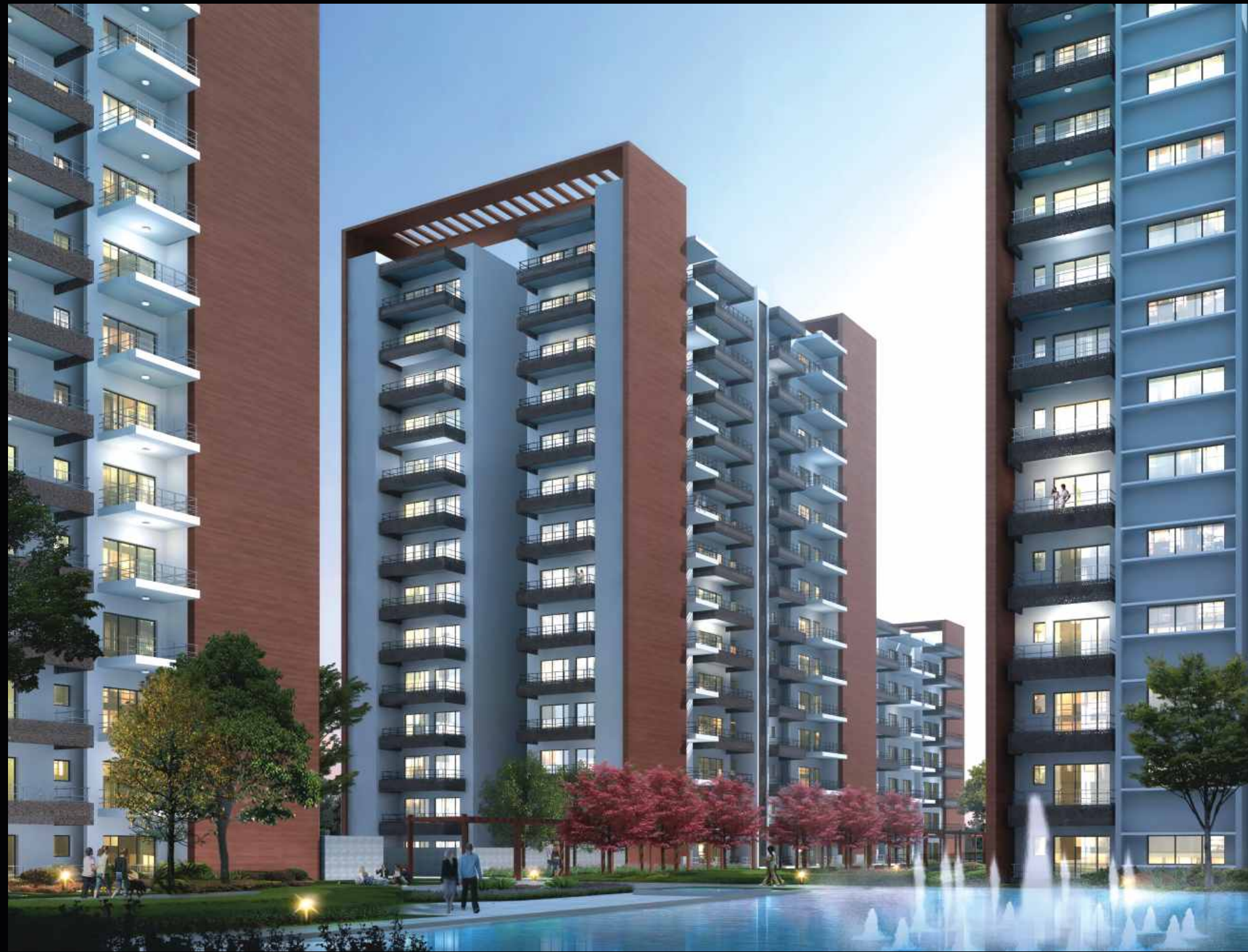
12 towers: spread across 12 acres with more than 75% of the apartments being 3- sides open
